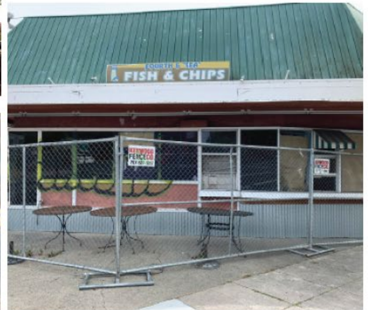
Abandoned Structure at 4th Street and C Street
